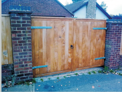
A gate, custom built to fit a between two pre-existing pillars.
