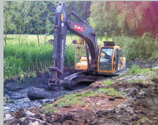
Excavating the boundary of a river.
