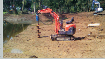
Boring the holes for fence posts.
