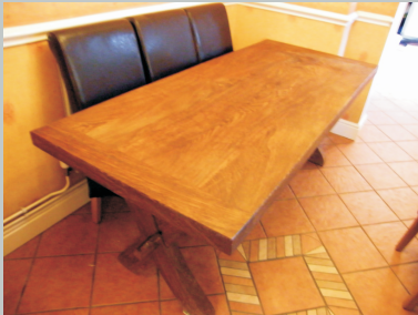
A dining room table, designed using traditional joinery (tusk tenons).
